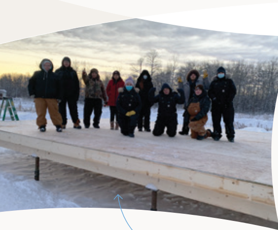
By December 17, 2020, the subfloor was completed.
