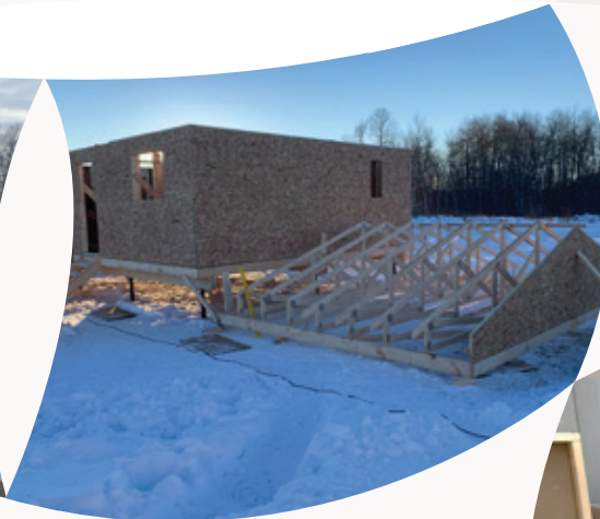
By mid-January, the ladies were putting on the roof trusses.
